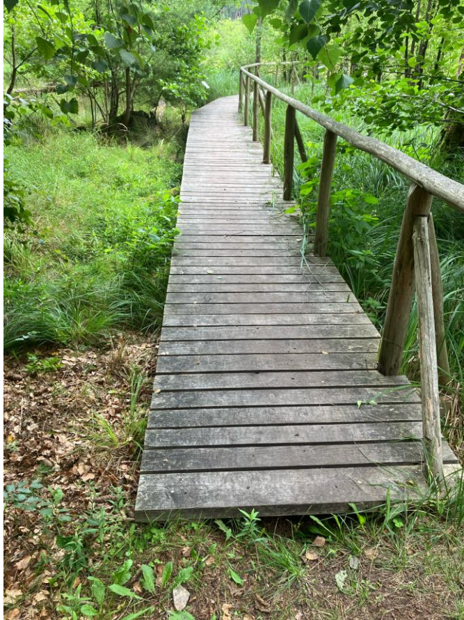
Fig. 11 The barrier-free facility in Wanderweg Serrah, to see the plants on the moor.
